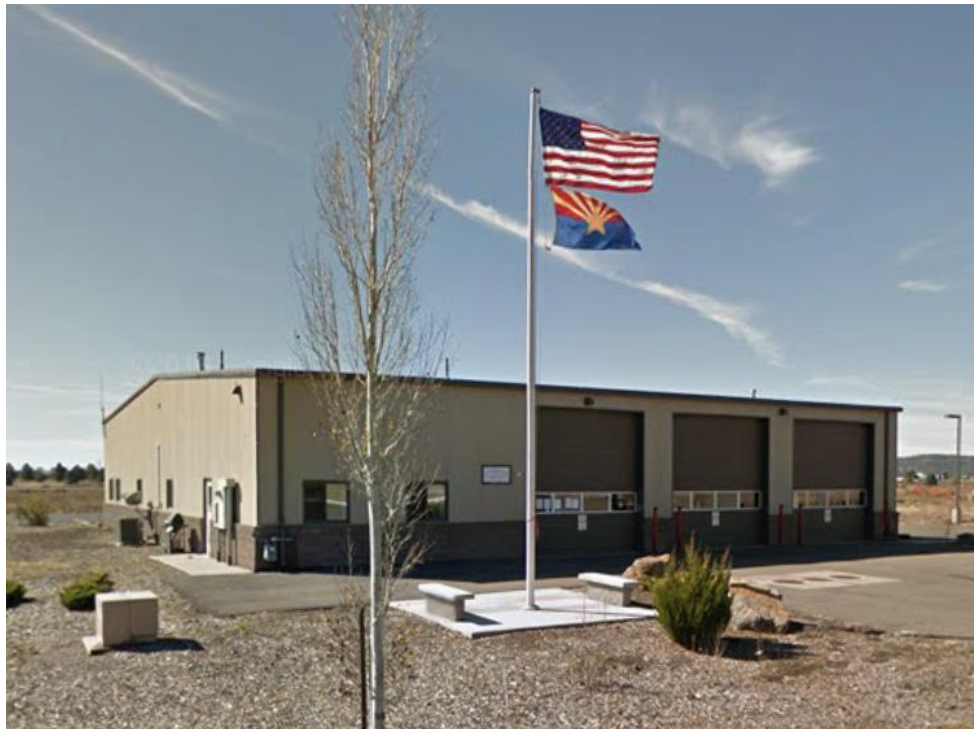
Figure 3: Street View of Existing Station
