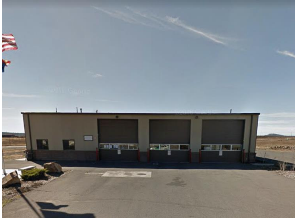
Figure 2: Front Face of the Existing Station
